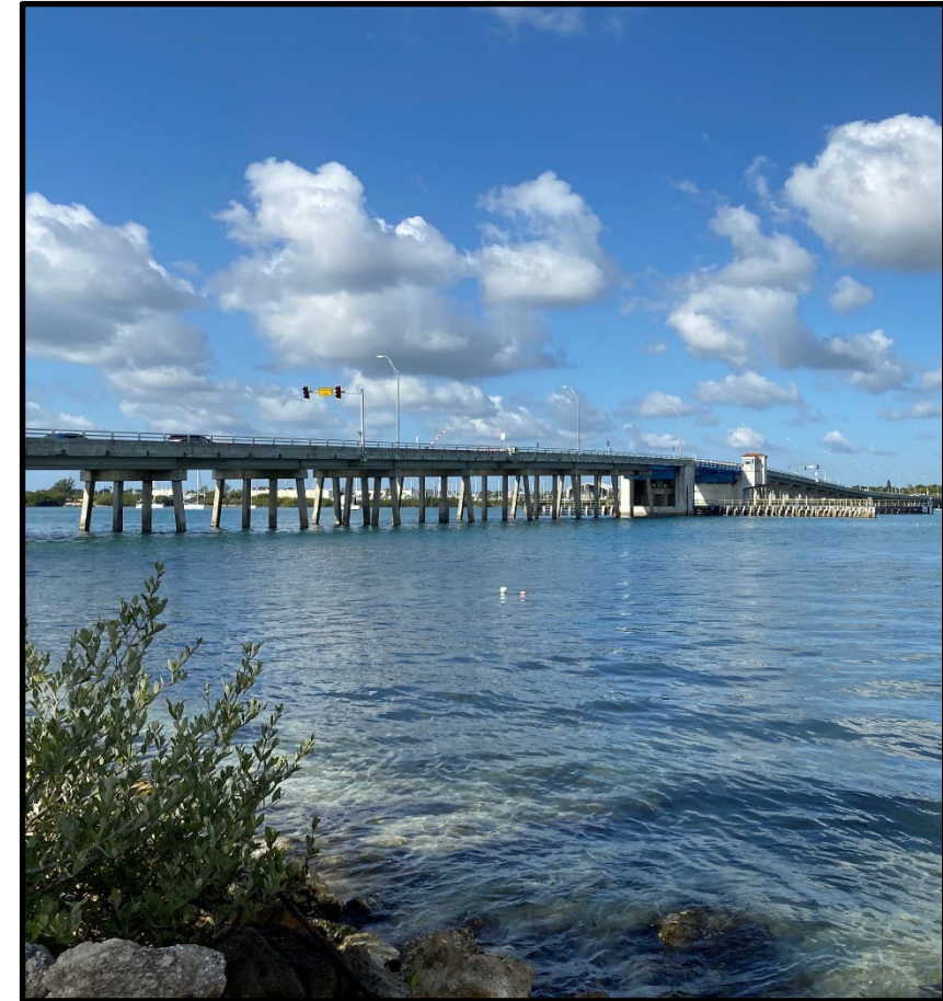
Existing bridge looking west (pre-construction)
