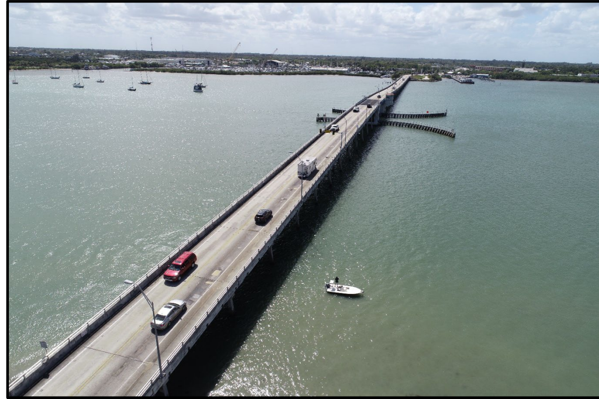
Existing bridge looking west. (pre-construction)
