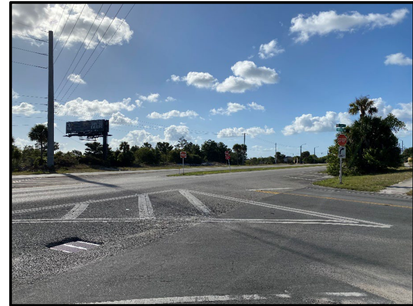
Intersection of Juanita Avenue and SR 5/US 1 looking south. (pre-construction)
