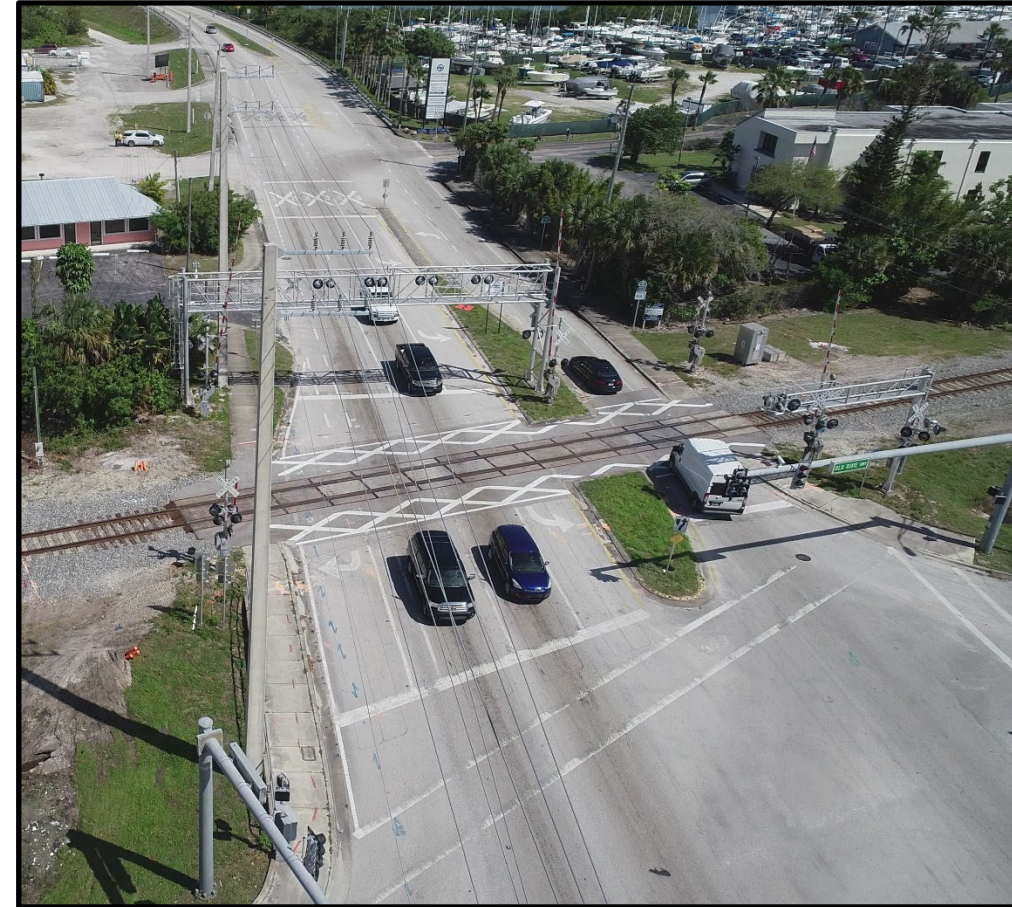
SR A1A looking east at the Old Dixie Highway intersection. (pre-construction)
